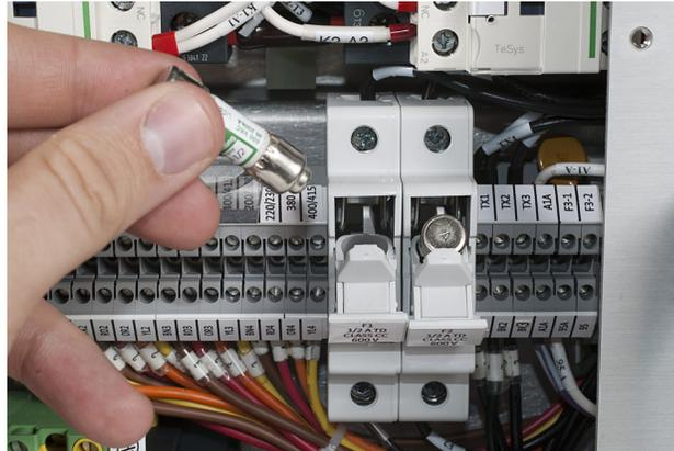
FIGURE 3-4 Fuses being inserted into the fuse holder
